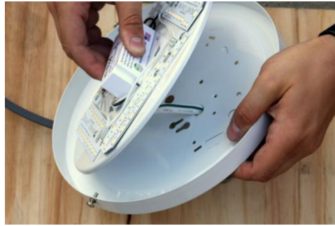
step 2: Bring LEDCR close to fixture pan. Route AC wires from LEDCR through a hole in fixture pan
